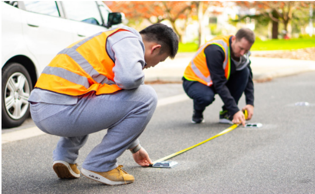
Installation is quick and easy. Taking the time to position sensors in a precise array ensures optimum data quality.
