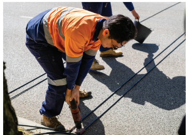
Installation is quick and simple on a variety of different road surfaces including gravel.
